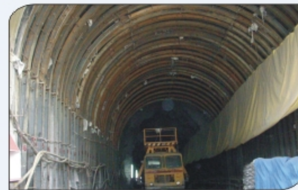
Bayal Adit of Rampur H.E. Project
