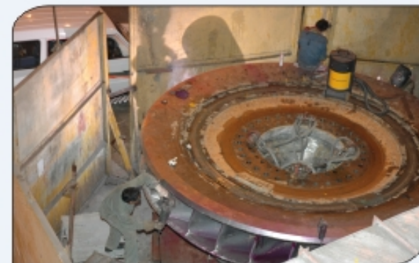
Runner Repair in progress at NJHPS
