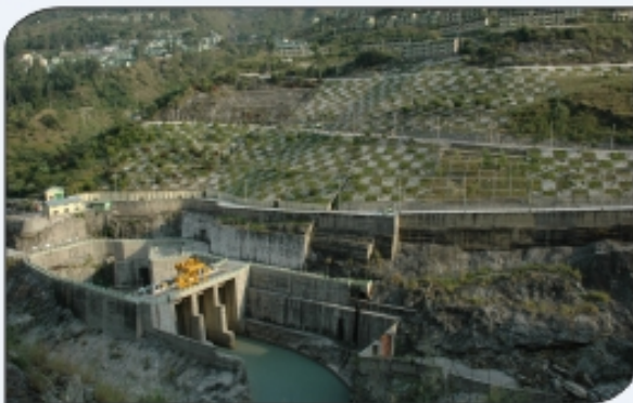
Outfall of the NJHPS with slope stabilisation & plantations
