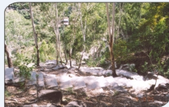
Construction of pucca paths in villages in the vicinity of RHEP
