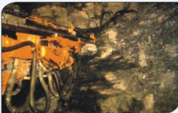
Drilling Operations at Kunni HRT
