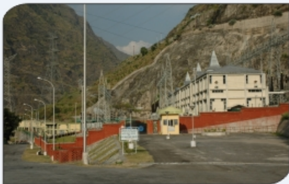
Power Transmission - Pot Head Yard
