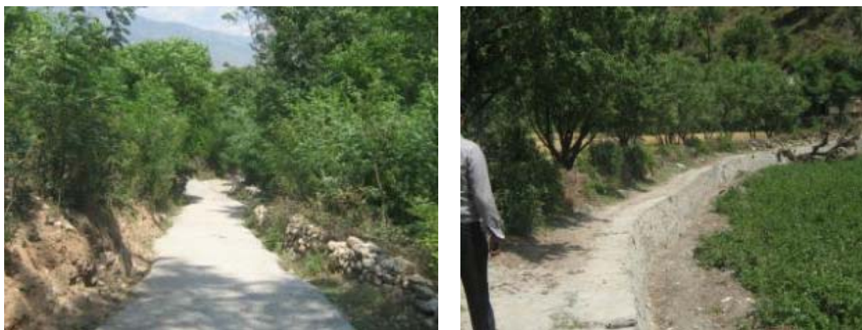
Photo 2.1 – An under construction Approach road and a Kuhl (irrigation channel) at Koyal village
