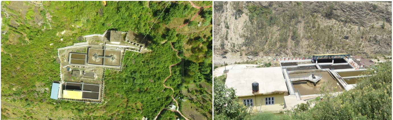
Ariel View of the Sewage Treatment Plant, Jhakri
