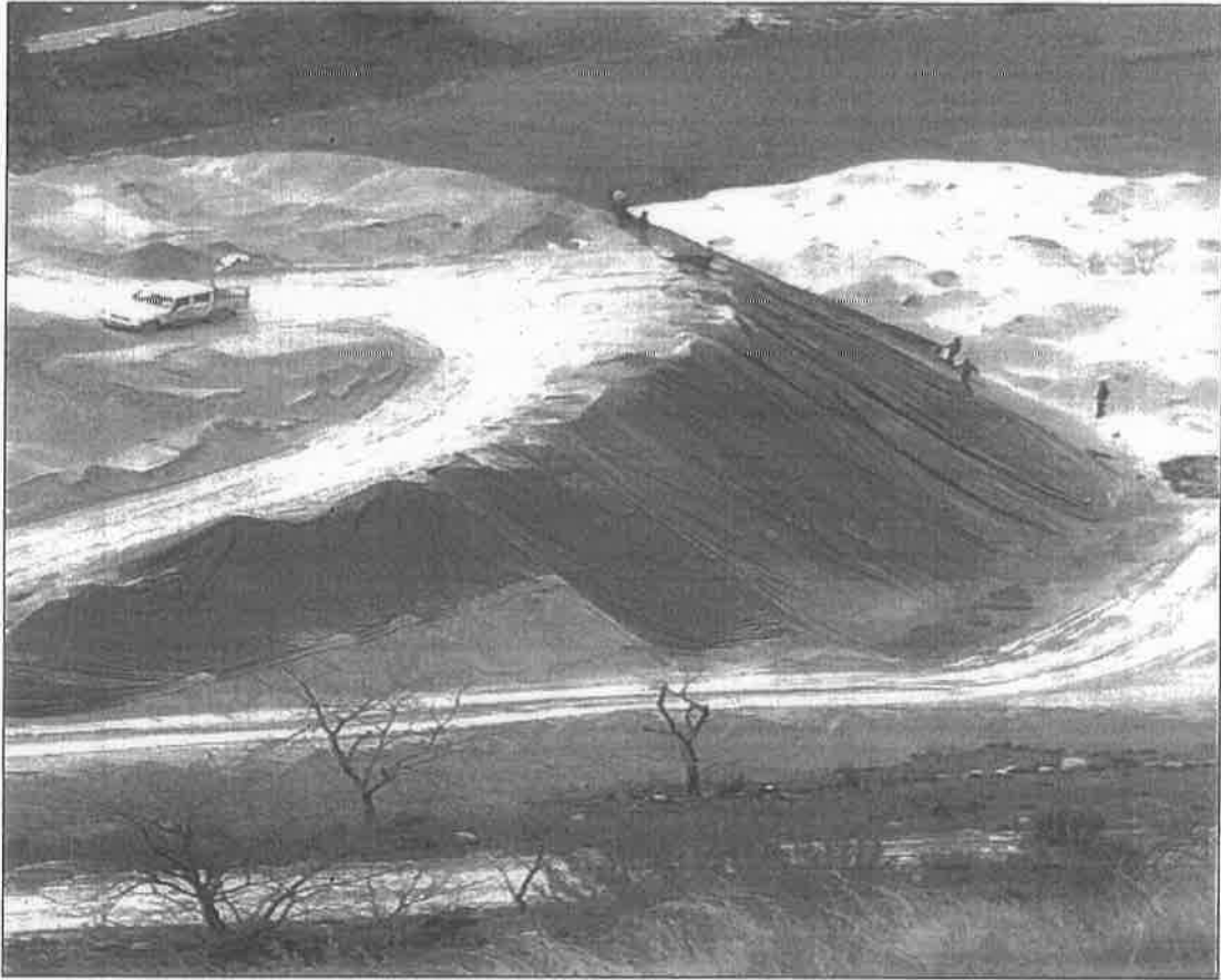
Picture-21. Crush material covered with trampoline to prevent dust emission.
