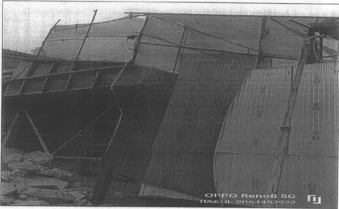
Picture-15. Crusher parts properly covered to prevent dust emission
