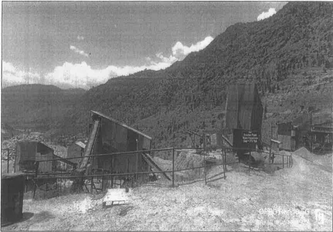
Picture-09. Crusher parts properly covered to prevent dust emission
