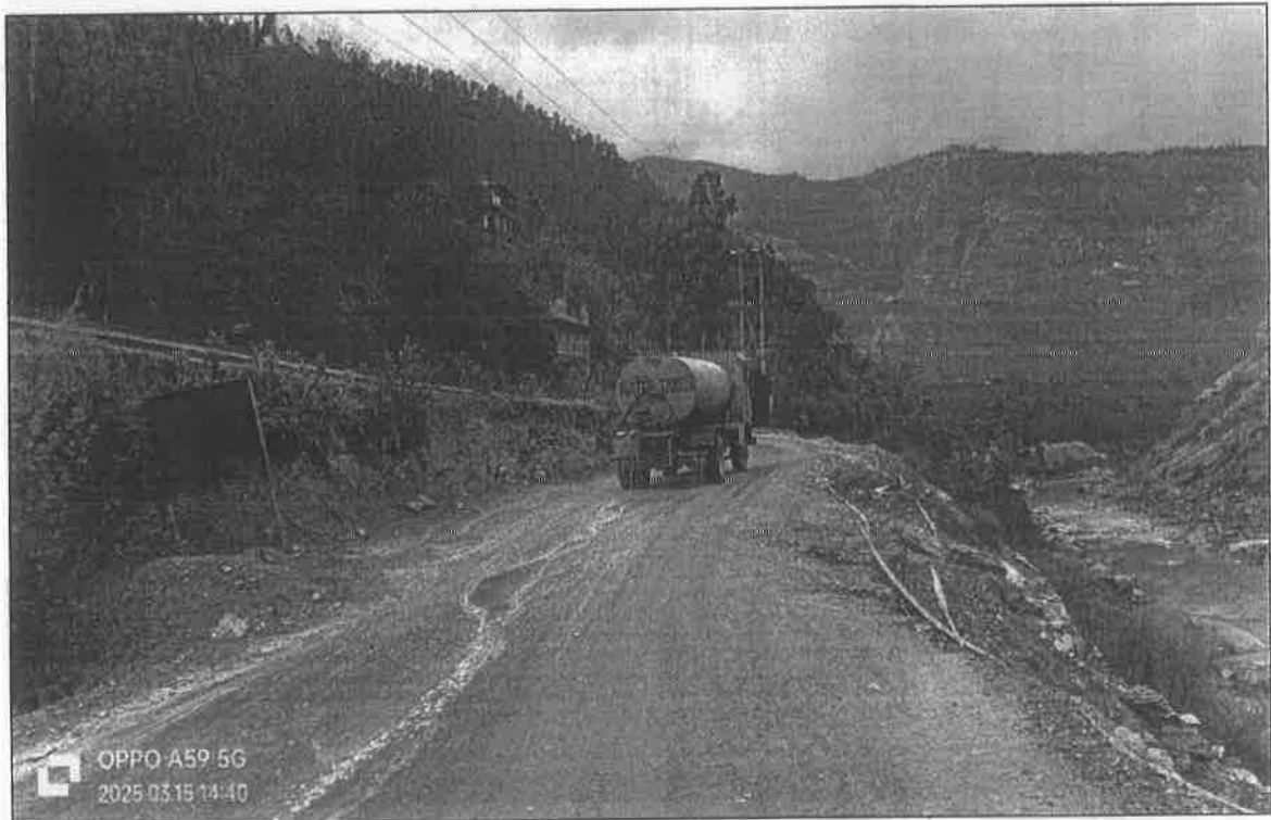
Picture-6. Water Tanker sprinkling water on site.
