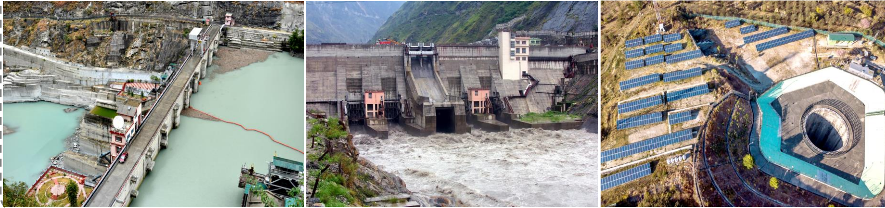
Nathpa Jhakri Hydro Power Station (NJHPS)
