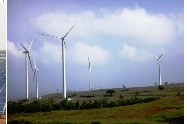
Sadla Wind Power Station
