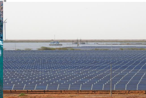
Charanka Solar Power Station
