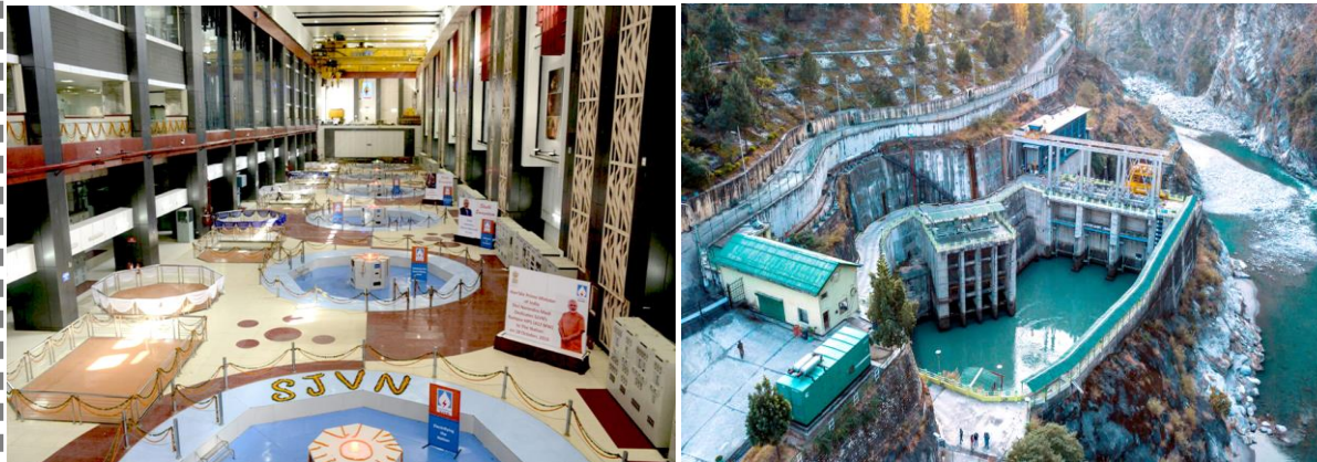
Rampur Hydro Power Station (RHPS)
