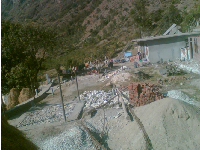
House construction works of PAFs is in progress in Bayal
