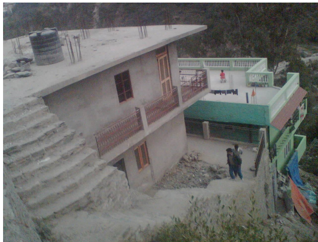
Newly constructed Panchayat ghar of Poshna Panchayat
