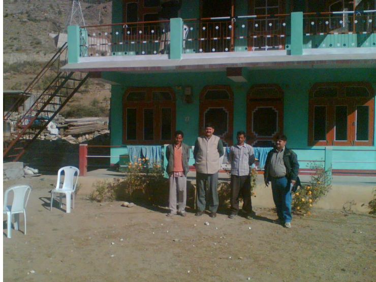
Monitoring team with the newly constructed house of Sh Govind Ram at Averi Village
