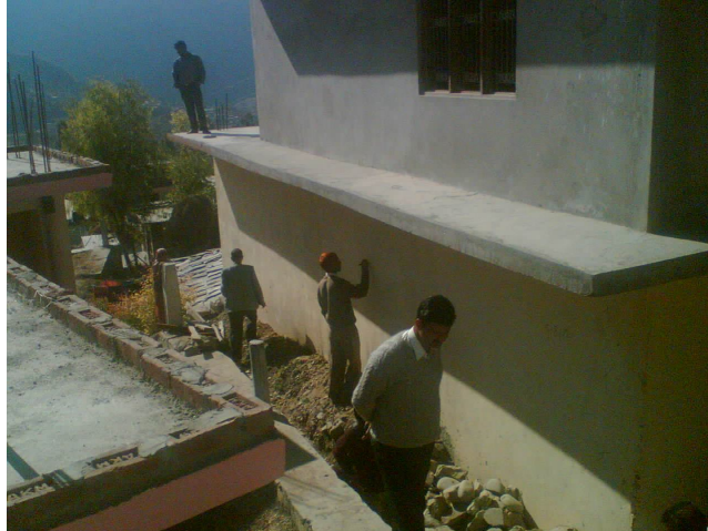
House crack checking committee marking houses at Bayal
