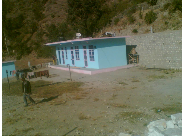
Newly constructed house of PAF at Bayal
