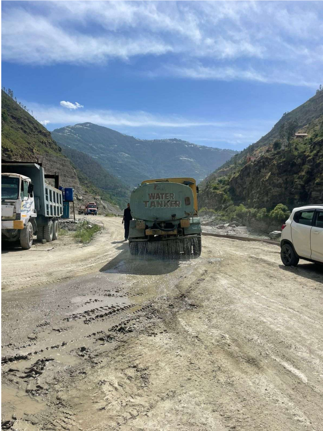
Water sprinkling is done throughout site.
